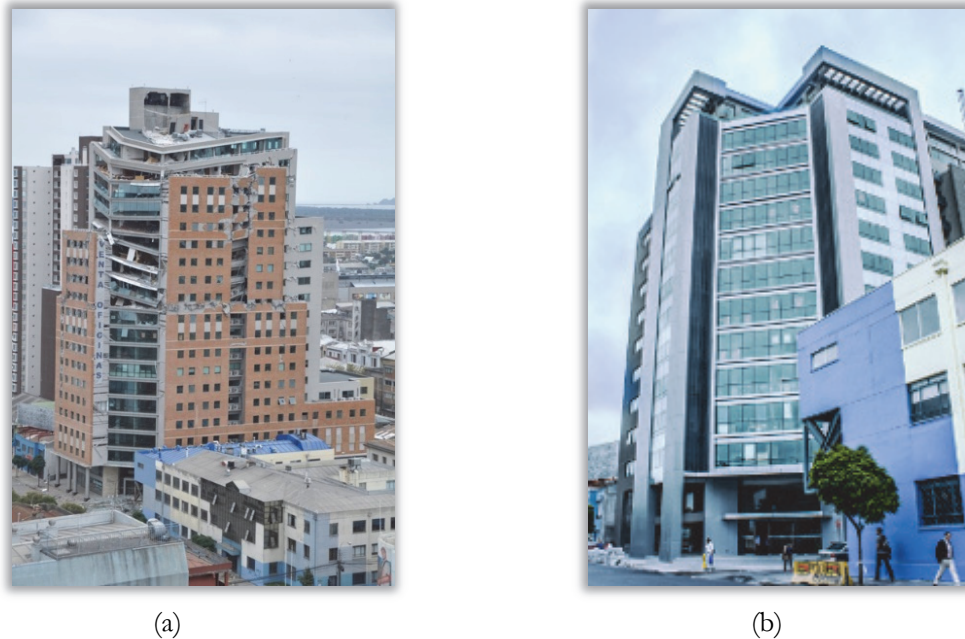
Figure 2-14. Torre O'Higgins building in Concepción, Chile: (a) building as damaged in the 2010 Maule, Chile Earthquake (photo courtesy of J. Harris) and (b) operational condition of the building ten years after the earthquake, parts of the originally constructed building were deconstructed (photo credit: Reid Middleton).
